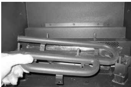
Burner Removed
