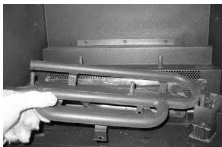
Burner Removed
