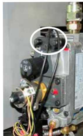
DC Sparker Wires
